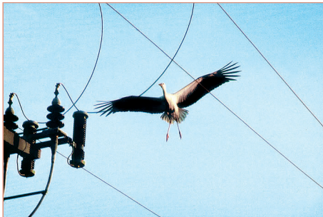
Stork landing on pylon © Manfred Loeffler
